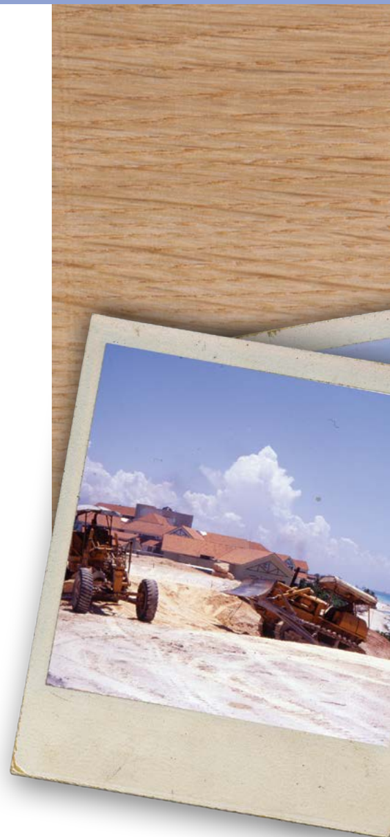
Shaping the grounds near the hotel complexes
