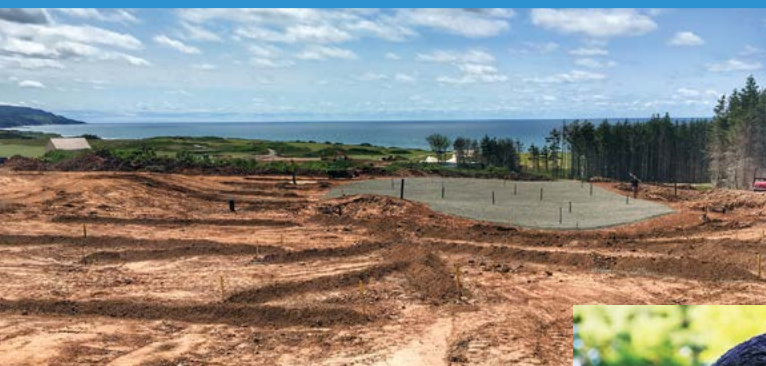
Drainage being installed on 10th green.
